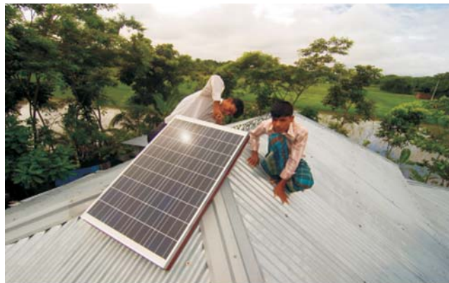
Figure - 1: A Solar Home System being Installed in Bangladesh
